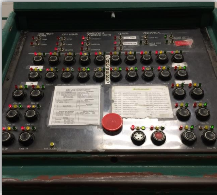
CB LIVING UNIT CONTROL PODIUM
